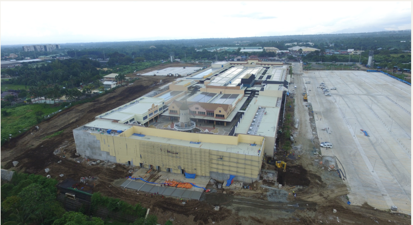
Acienda taking shape during construction, September 2018.
